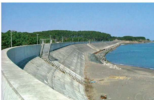
Sea wall with stairway evacuation route used to protect a coastal town against tsunami inundation in Japan. Photo courtesy of River Bureau, Ministry of Land, Infrastructure and Transport, Japan.
