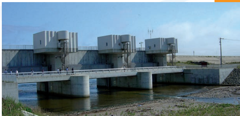
Water gate used to protect against tsunami waves on Okushiri Island, Japan. The gate begins to automatically close within seconds after earthquake shaking triggers its seismic sensors. Photo courtesy of ITIC.
