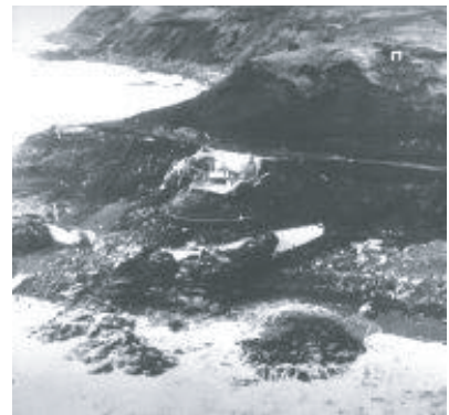
Scotch Cap Lighthouse before (above) and after a tsunami in 1946.
